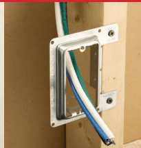
Mounting Plate Bracket MPLS
