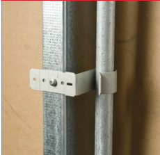
Screw-on Conduit Support CS812 & CS812D
